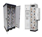
Minimum cabinet height = Rack height (to top of rail) + Battery height + Space above battery (12" ideal) + Charger height + 6" (for space above charger) Calculating Cabinet Height Chargers need room to breathe and batteries need extra room above for maintenance (watering and testing).
