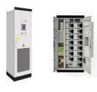
BMS plays the role of perception in the energy storage system, and its main function is to monitor the operating status of each battery in the battery energy storage unit to ensure the safe operation of the energy storage unit.
