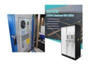
Battery Energy Storage Systems (BESS) Definition. A BESS is a type of energy storage system that uses batteries to store and distribute energy in the form of electricity. These systems are commonly used in electricity grids ???
